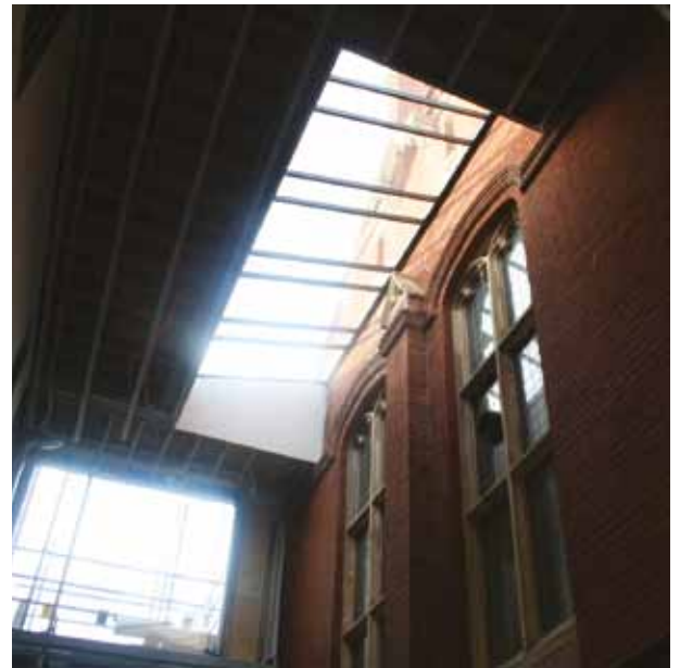
November 2016: Looking up at the atrium skylight
