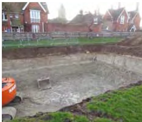
December 2015: A large hole appears at the edge of College Field; not the new swimming pool, but preparations for a 'soakaway' to cope with waste water from the new building
