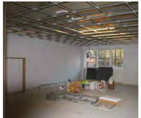
November 2016: One of the new classrooms being fitted out
