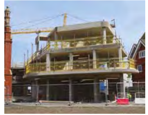
June 2016: The outline of the three-storey pavilion becomes clearer
