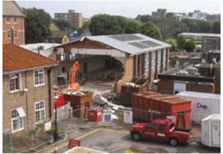
In 2015, a similar view mid-demolition
