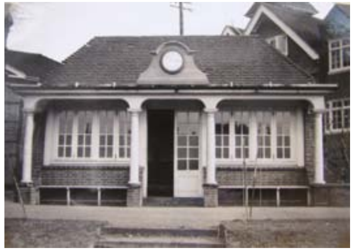
Extended in 1931 with glass windows and doors; the clock was added in 1939
