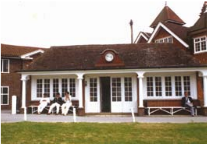
This view from the 1970s shows the expansion work of 1969; the doors are wider and there is an extra panel in both windows
