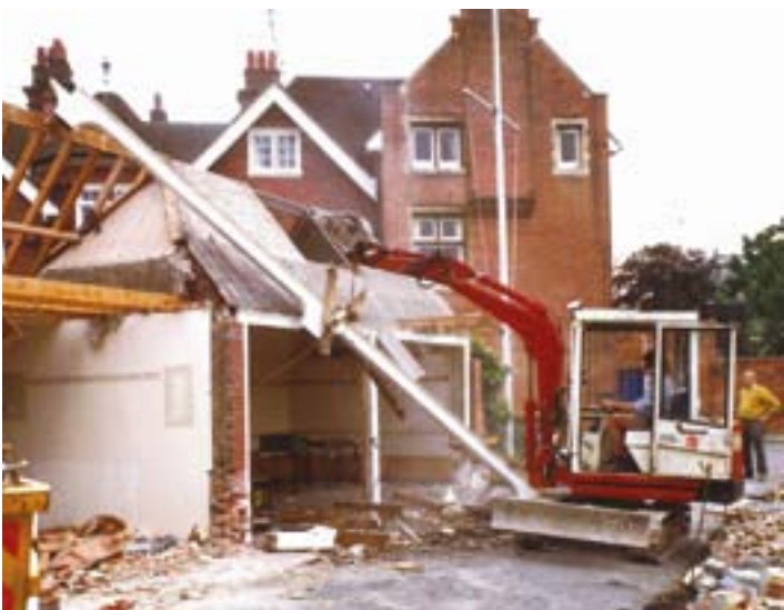
The demolition in 1993
