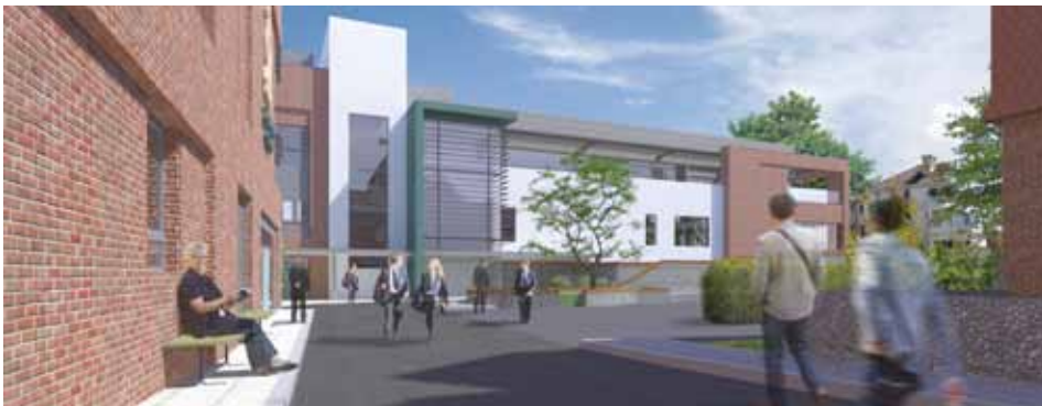
The Eastbournian Society will be playing its part as the College embarks on the Project 150 development (artist's impression)
