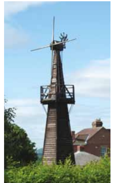
The tower of the Castle Fruit Farm Windmill erected at Dymock in Gloucestershire still stands although the sails and fantail are gone. Further mills were erected on the Westward Islands and at Blackheath near Guildford
